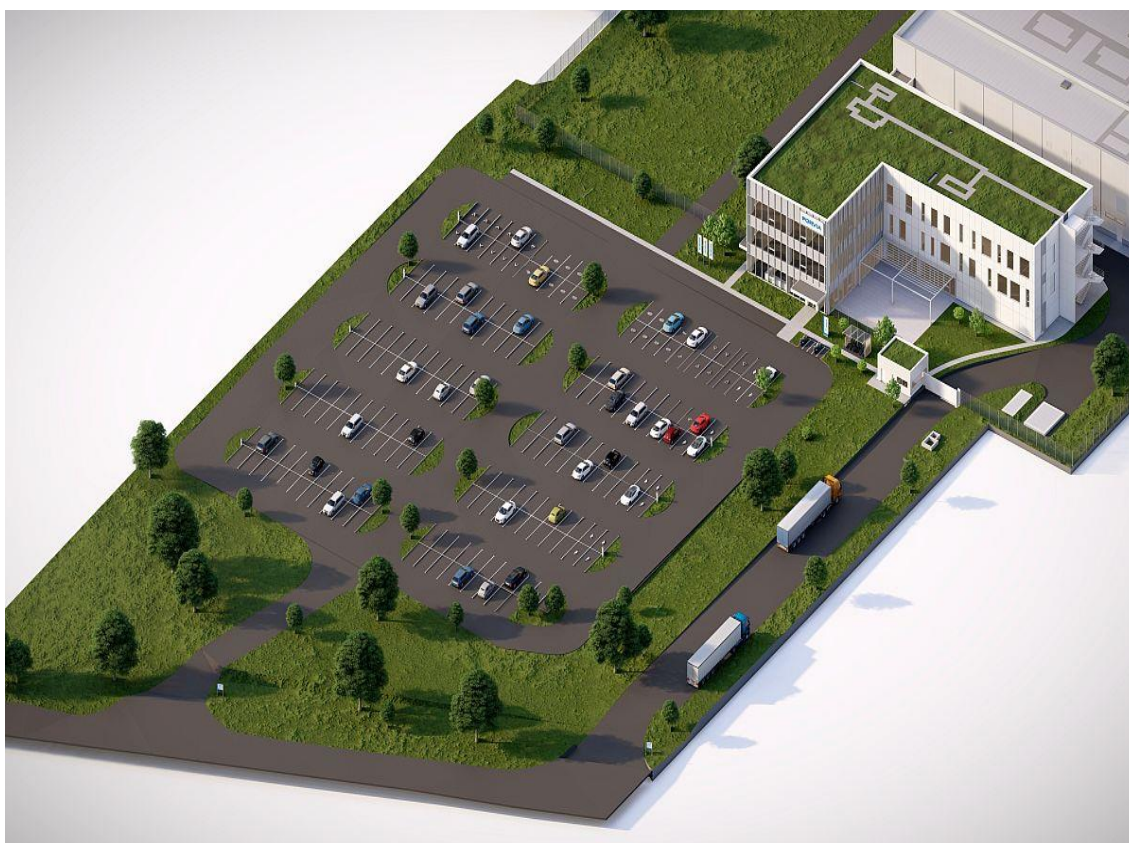
Figure 5-2_HELLA new building, which will be climate neutral by 2025
