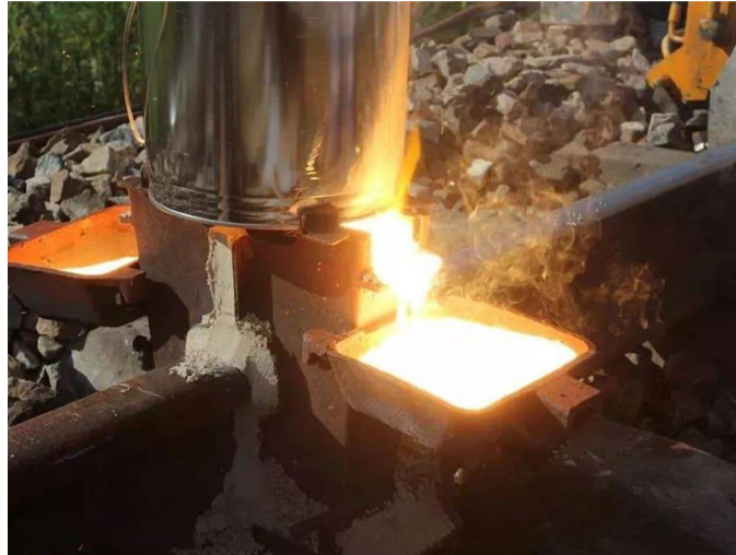
Figure 32. Railway track thermite welding [28]
