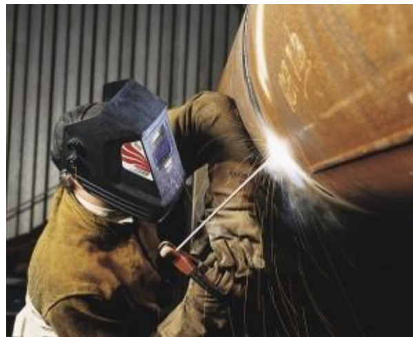
Figure 38. Manual metal arc welding [32]
