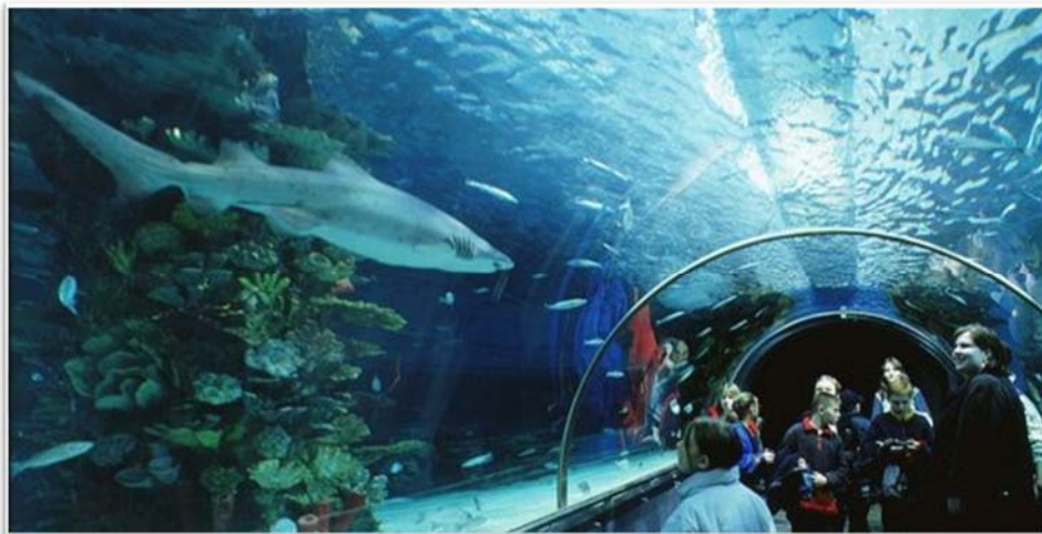
The glass tunnel of the Tropicarium in Budapest is a good example for an externally loaded pipe
