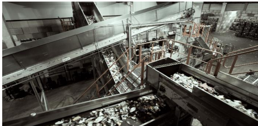
4-6. Figure_ Belt conveyors [18]
